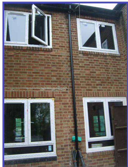
Figure 7. property has now been refurbished using grant funding
