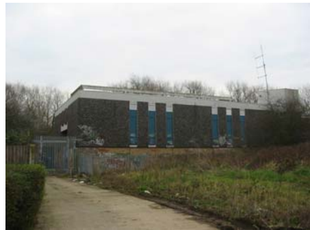
P7: Former Electricity Sub Station
