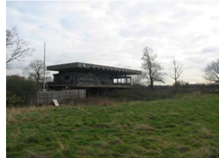
P11: Derelict Pavilion (northern boundary)
