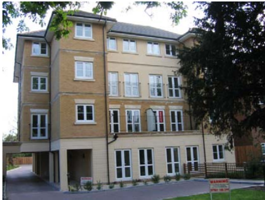
P16: 13 Copers Cope Road, Beckenham
