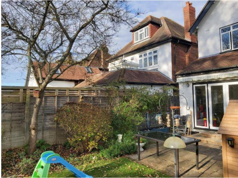
Photo 3. View towards rear of No. 39 Wood Ride.
