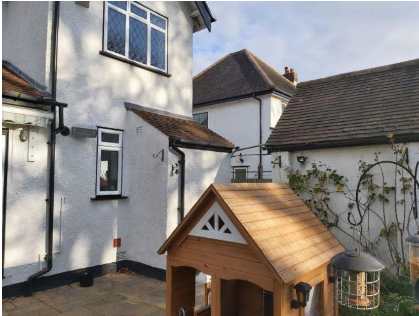
Photo 4. View towards rear of No. 35 wood Ride.
