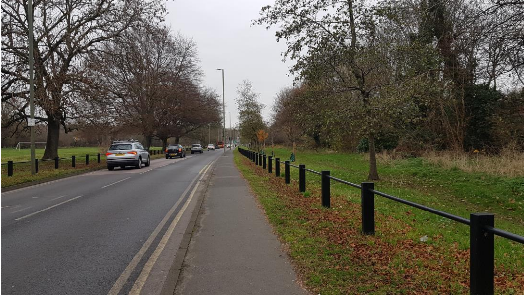
Photo 1. Application site surroundings looking north.
