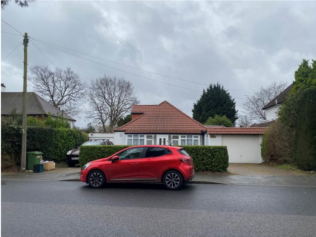
Figure 4: Photo of Front Elevation:
