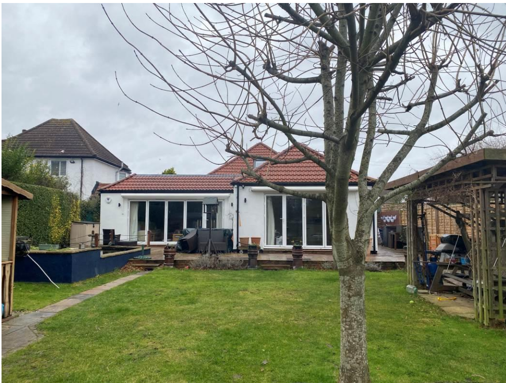
Figure 5: Photo of Rear Elevation
