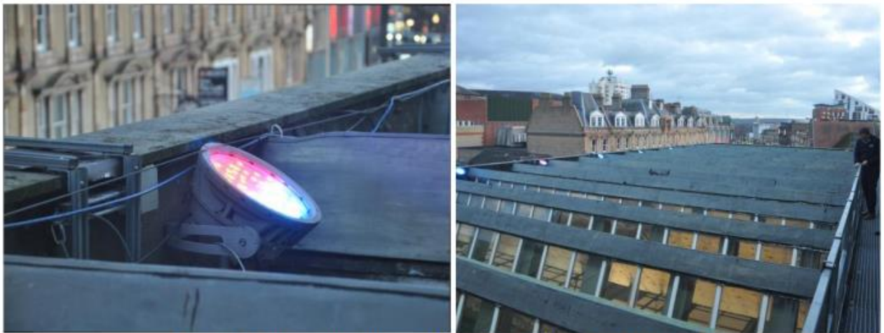
Figure 4: Existing Luminaires on the First Floor Roof will be Removed
