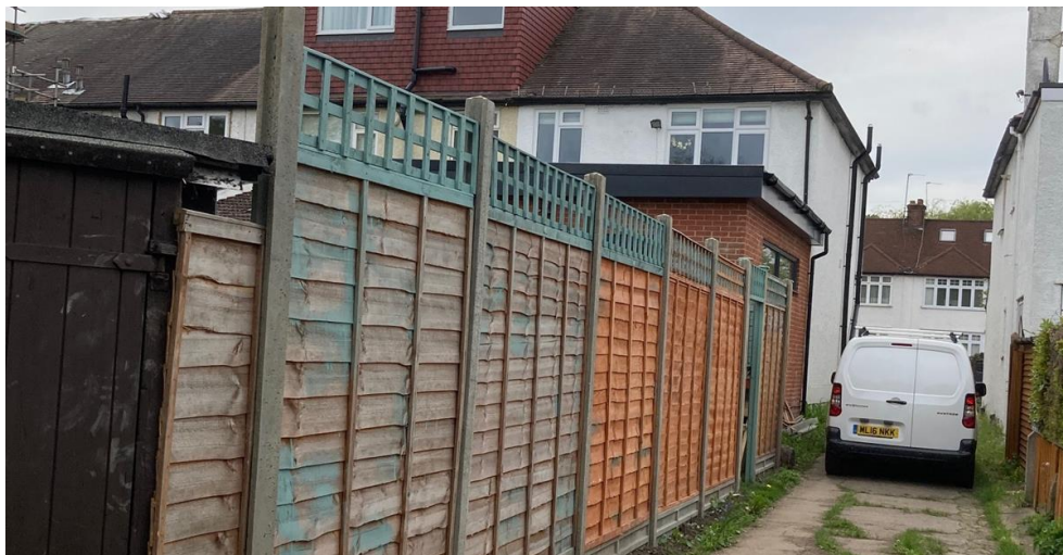
Photograph 2: View from access
