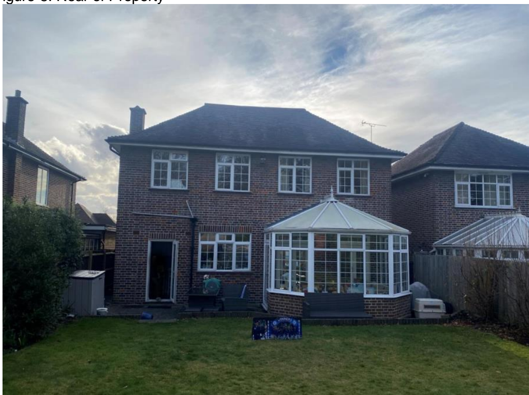
Figure 5: Rear of Property
