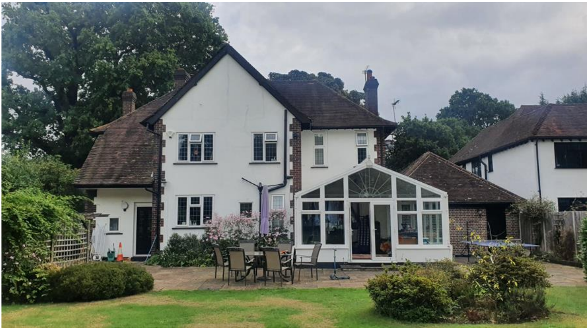
Fig.3 – Site photo (Rear)
