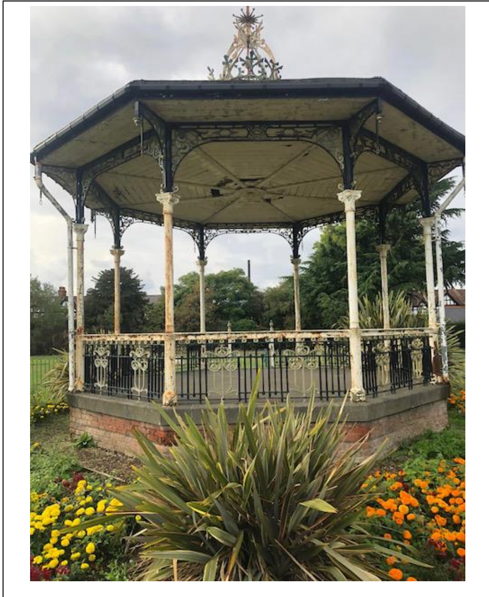
Figure 3: Photograph of existing Bandstand
