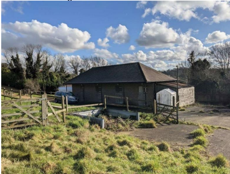
2.1.5 Photo 1. Existing stables viewed from north west.
