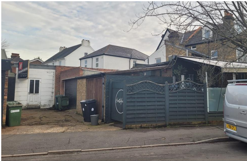
Figure 3: View of Rear Access
